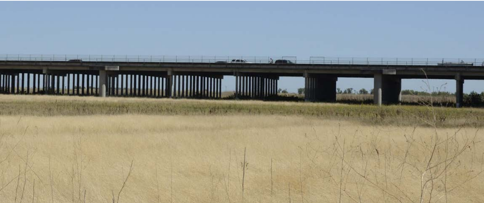
Concrete slab bridge causeway
