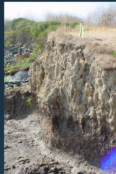
Eroding levee along San Pablo Bay
